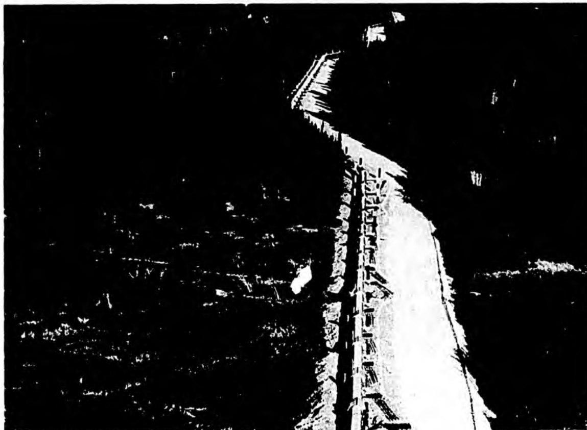
A portion of elevated pipeline snakes its way along the 800-mile route from Prudhoe Bay on the Arctic Ocean to Valdez in south central Alaska.
