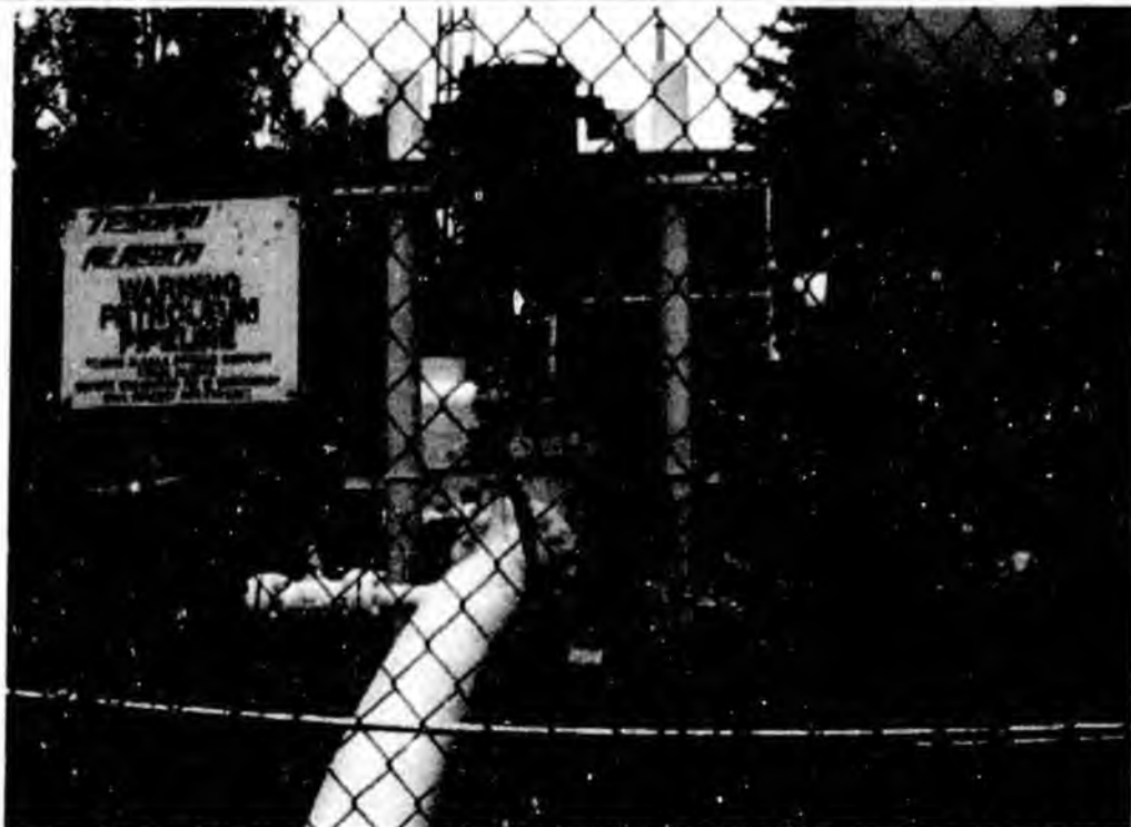
This photo is of a remotely-operated valve on the Nikiski Alaska Pipeline near Point Possession. Solar panels and propane provide energy for the valve and cathodic protection system.
