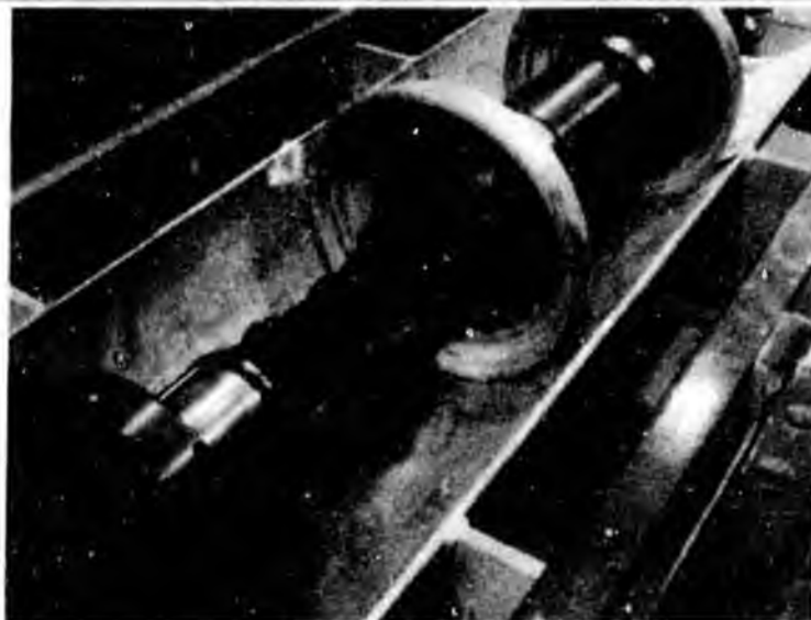
This smart pig was used in June 2005 to detect pipeline conditions in the Alpine Oil Pipeline. The lease compliance oversight team witnessed retrieval of the pig at Kuparuk.
