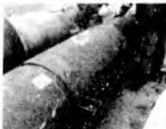
Line leak and sleeve installation
