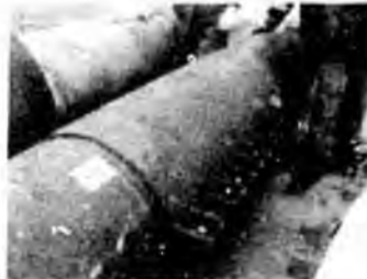
Line leak and sleeve installation
