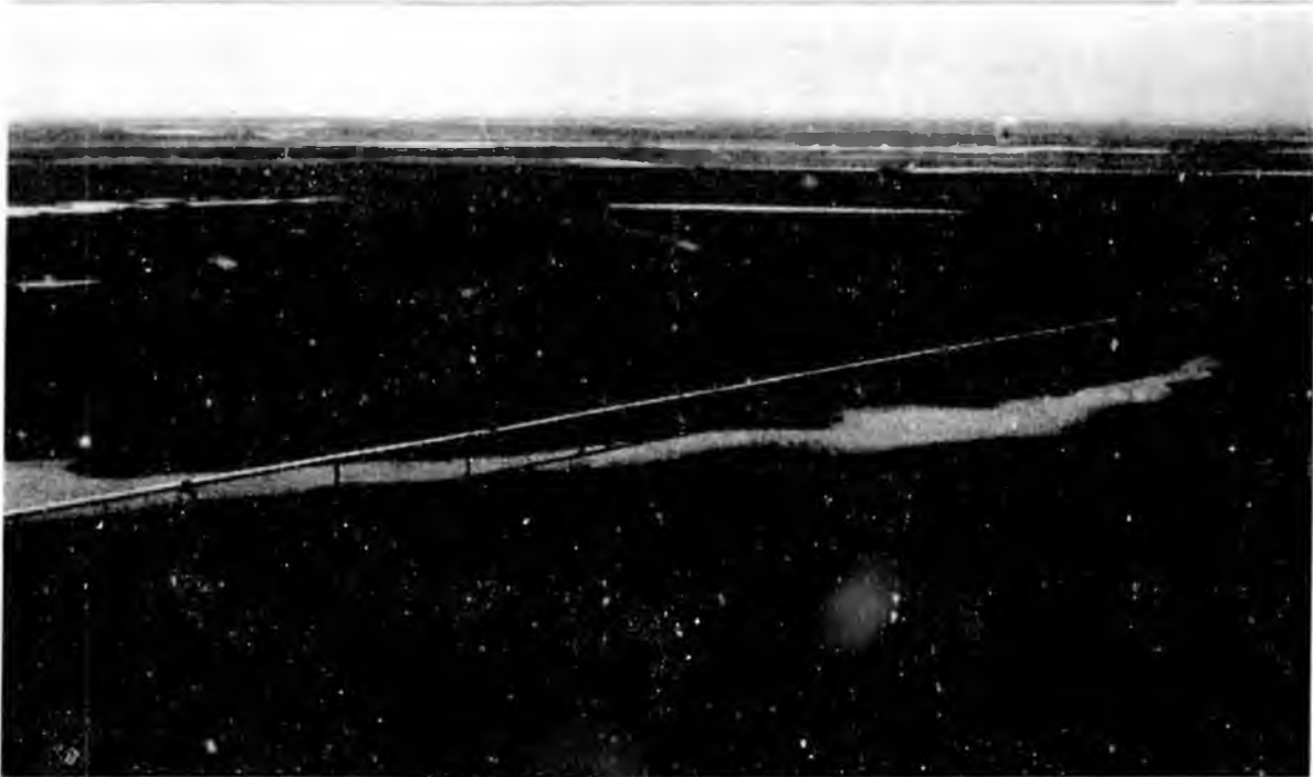
The Badami pipelines cross were built "roadless" to prevent damage to tundra.
