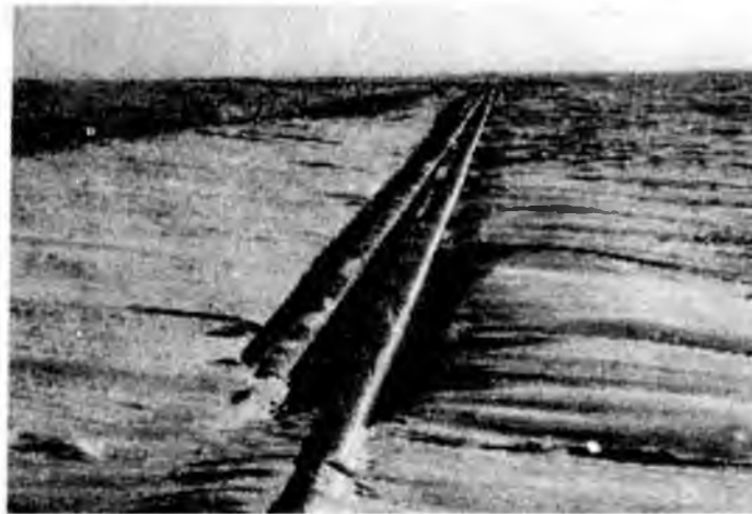
Winter view of the Milne Point Pipelines looking South from the "S" Pad intersection.
