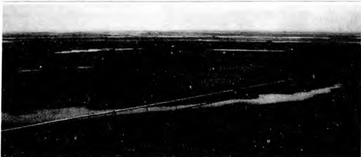
The Badami Sales Oil Pipeline transports processed crude oil from the Badami Development on the east to the Endicott Pipeline. The Badami Utility Pipeline, resting on the same supports, has been used to transport fuel gas from Endicott to Badami.
