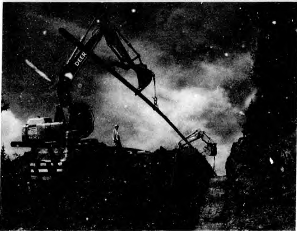
In summer 2006, construction is in progress on the 4.2-mile Kasilof Extension to the KKPL. This picture shows a segment of pipeline being placed in the newly-dug trench.
