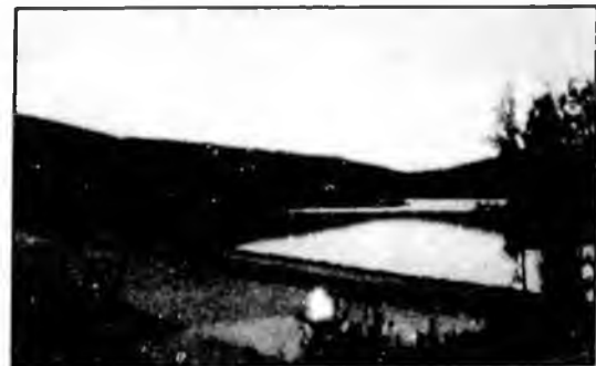
The Fort Knox tailings dam is the largest earthen dam in Alaska.
