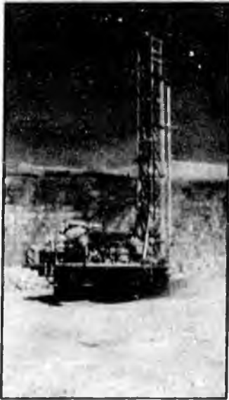
DR7 drills holes on a new blast pattern at Fort Knox.
