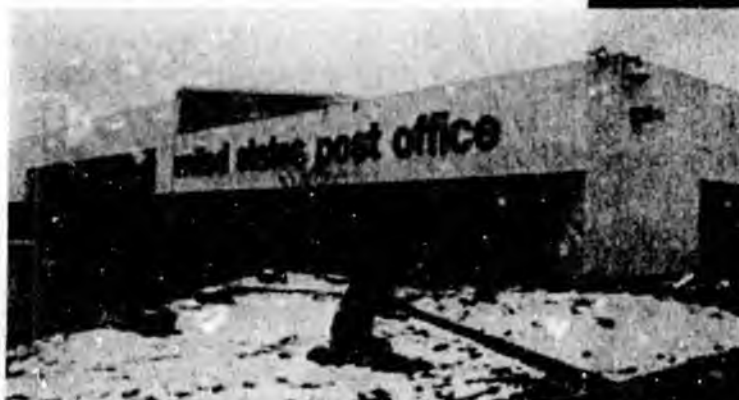
The Mail Processing and Distribution Facility, adjacent to the Anchorage International Airport, is key to the Alaska mail system.
