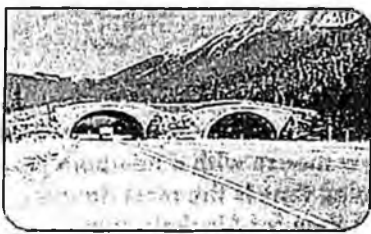
Overpass proven highly successful for moose crossing over railroads or roads.
