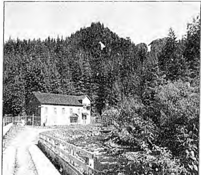
Taken out of service in 1998, this is one of two power houses built to generate power that used water from the Salmon Creek Dam. Photo is courtesy of Alaska Electric Light & Power Company.
