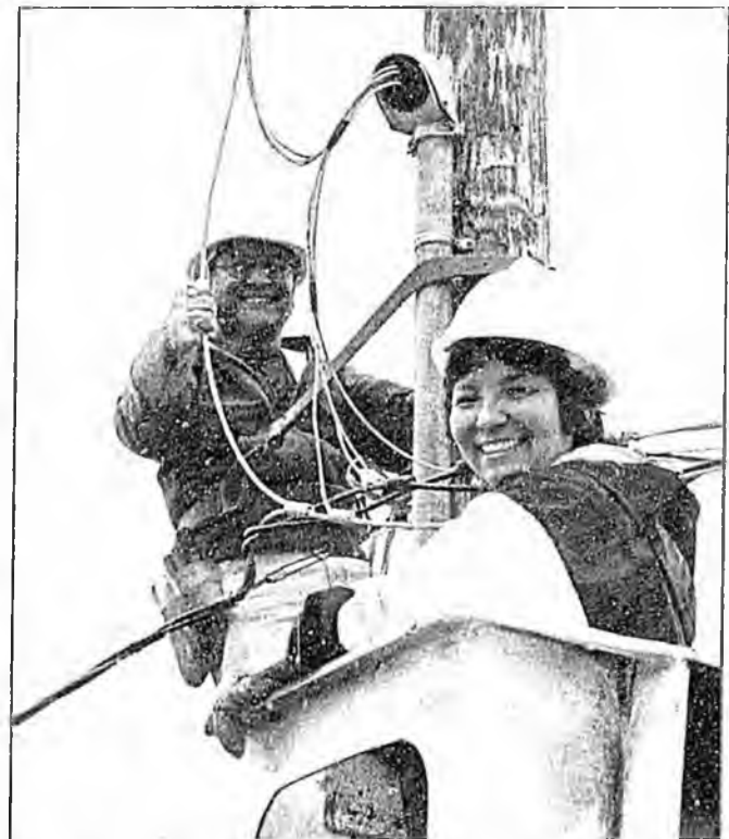
Alaska Power & Telephone Company (AP&T) Metlakatla crew (Richard Booth and Kathy Brendible) are shown working on a power pole. Photo is courtesy of AP&T.
