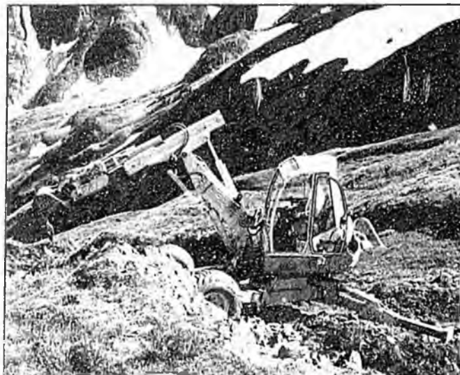
A "Menzi muck" machine carves out a trench to bury power lines. Photo is courtesy of Alaska Electric Light & Power Company.
