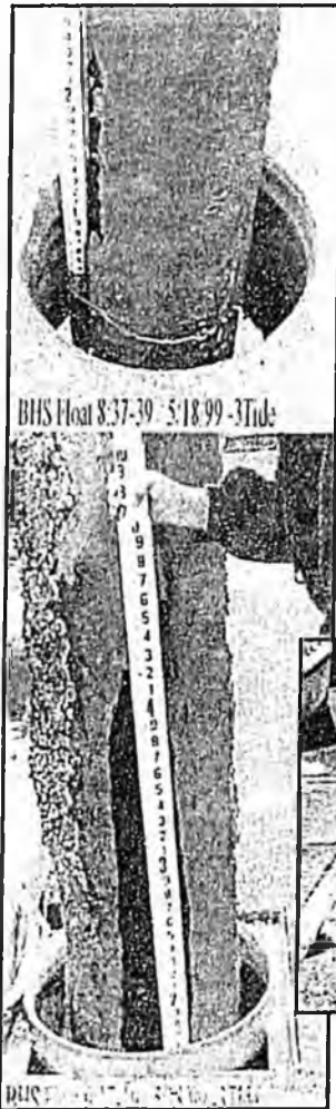
Above: Concrete damage at Valdez Harbor Left: Damaged Harbor Piling
