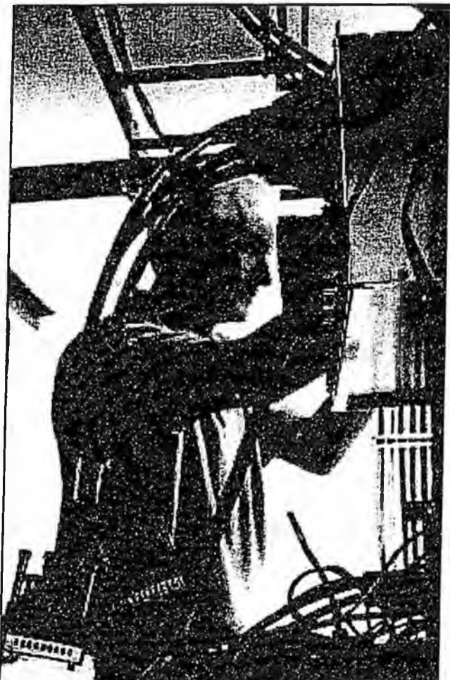
Manager of Alaska Power & Telephone Co. (AP&T), Wendell Hewes, works in the Wrangell Central Office. Photo is courtesy of AP&T.
