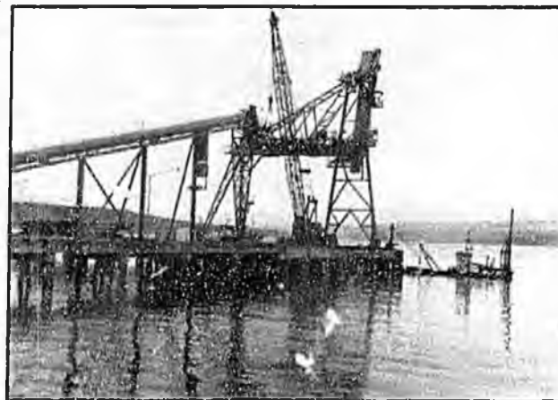
The Homer Deep Water Dock and the chip-loading conveyor superstructure used to load chip ships bound for overseas ports.
