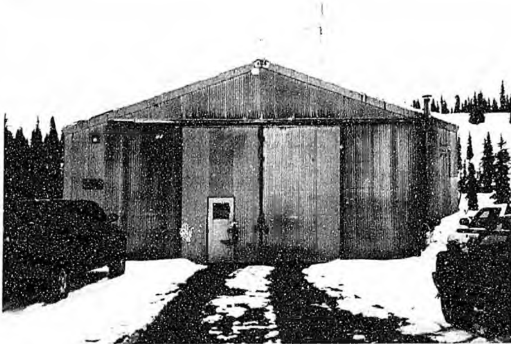
Photograph One: Maintenance Shop as viewed from the East
