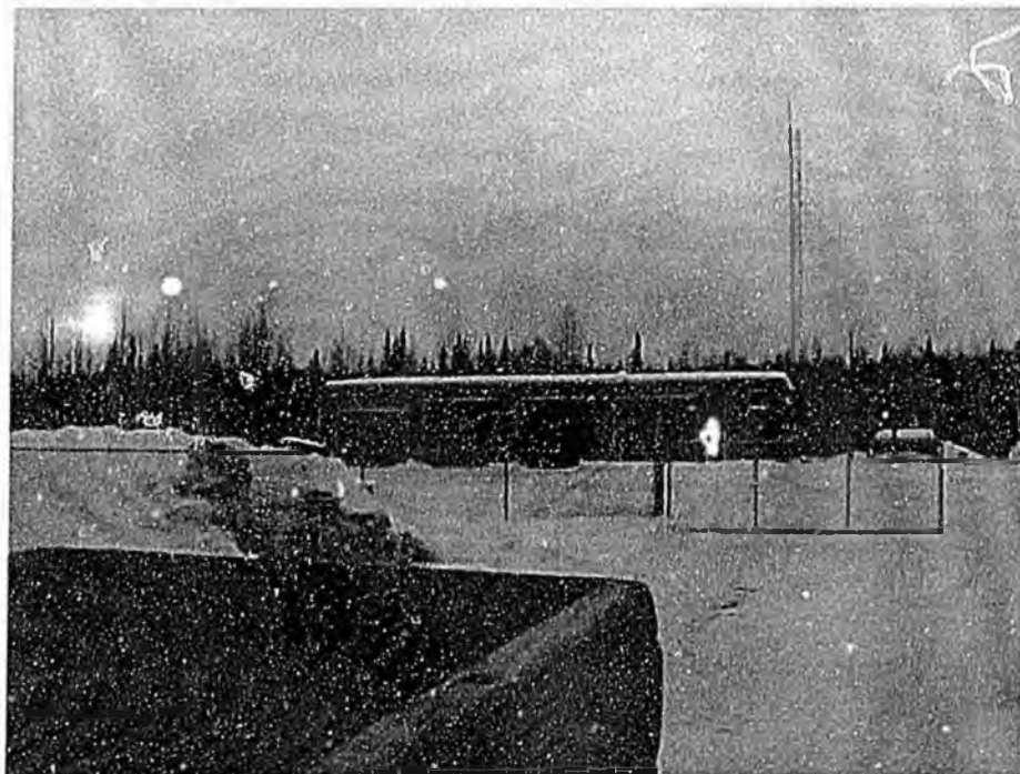
Photograph Two: Maintenance Shop as viewed from the Parks Highway
