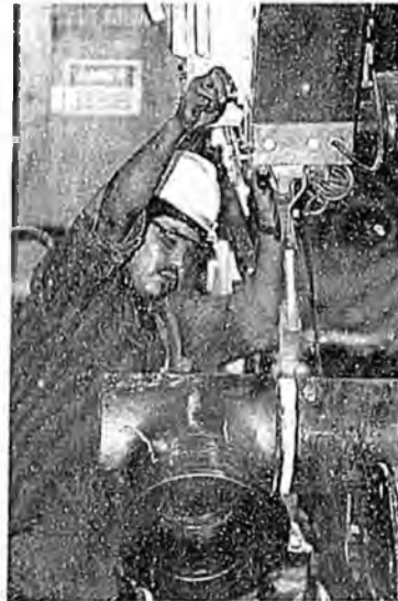
Pipe fabrication for BP's Northstar project in Anchorage
