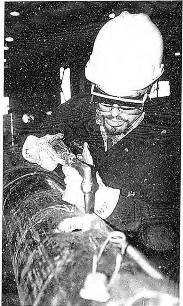
Fabrication under way at Natchiq's plant in Anchorage.
