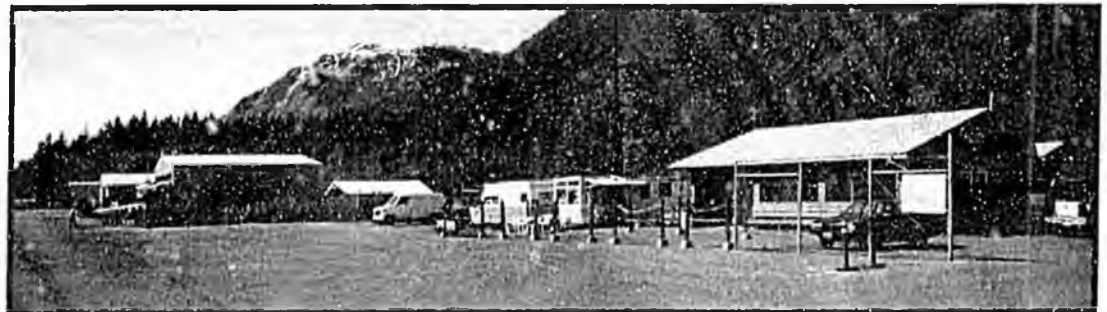
Haines airport, part of the territory annexed to the City of Haines in 1999.
