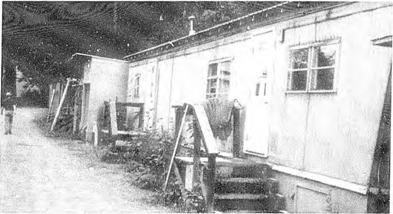
Trailers continue to house some administrative and maintenance operations.
