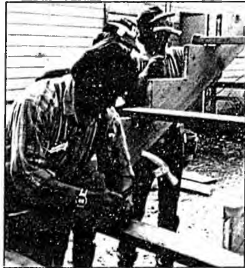
Brady Wallis and two co-workers construct steps to the shed.
