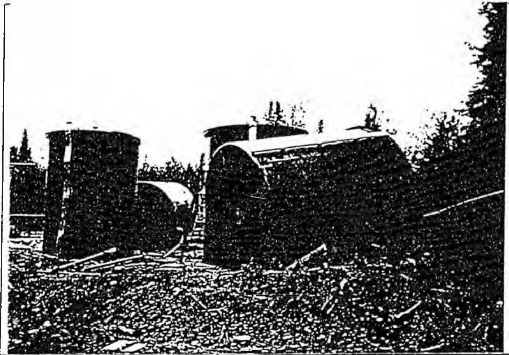
Photograph A.13 Tank farm located within a flood plain. Tanks tipped over and facility severely damaged by flood.
