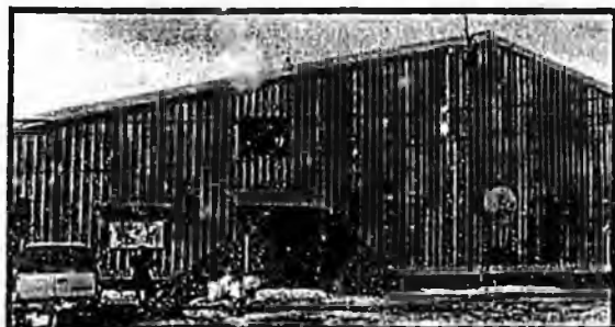
Akiak Community Building
