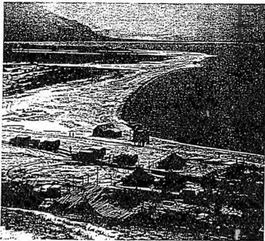
Corps of Engineers camp on the shore of Kluane Lake. This photo was taken in the early morning when trucks lined up to take troops to work. Note logs in foreground used to build "corduroy road" over permafrost.
