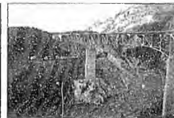
△ The Alaska Railroad crosses the trestle near Denali National Park.
