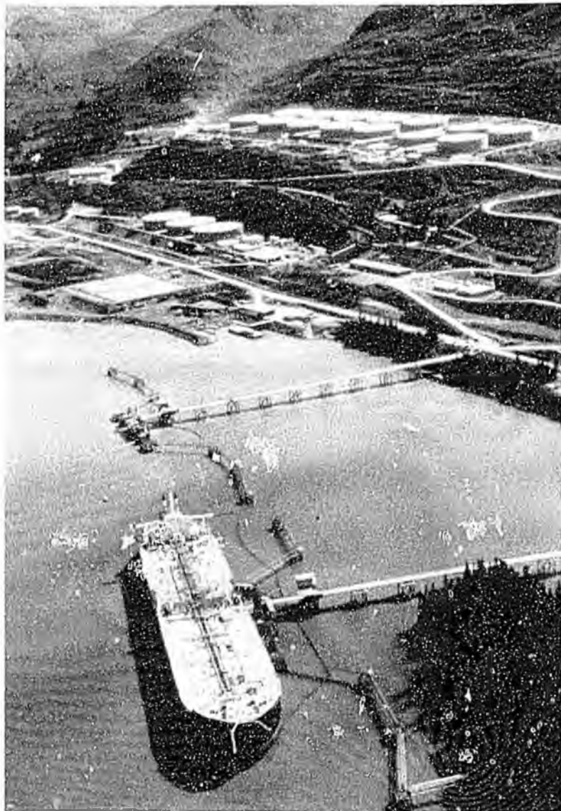
Terminus of the Trans-Alaska Pipeline in Valdez, Alaska.
