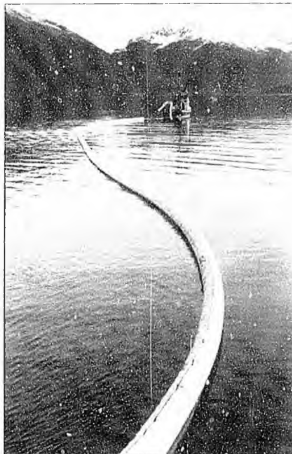
Fishing vessel tows boom during a spill drill. Local fishermen demonstrated in 1989 that they could be effective components of spill response.
