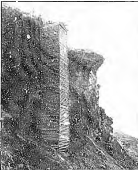
Figure 38. Cribbed shaft exposed in Fish Creek drainage, Fairbanks district, during overburden removal. In early days, hundreds of these shafts penetrated the deep frozen overburden of the Fairbanks district in search of rich, but deeply buried, placer gold deposits. (Photo by Bob Tsigonis)
