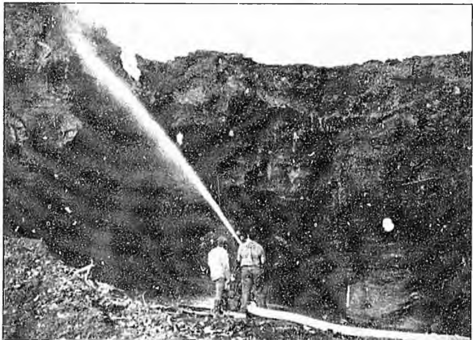
Figure 39. Hydraulic removal of overburden at Shoreham Resources' Tofty operation, Hot Springs district. This time-tested method can still be used to efficiently move overburden, provided effluents are contained and water quality maintained. (Photo by Shoreham Resources)
