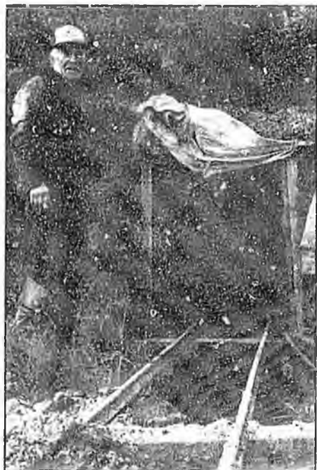
Figure 32. Jack Hoogendorn inspects the entrance to his underground drift mine on the right limit of the Innachuk bench in the Innachuk district near Deering on the Seward Peninsula. Jack covers the entrance to prevent the frozen gravels from thawing and caving during summer months. (Photo by T.K. Bundtzen)
