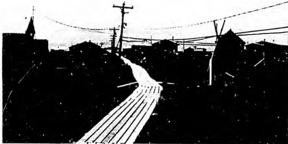
Photograph 3: Low clearance and leaning pole over boardwalk
