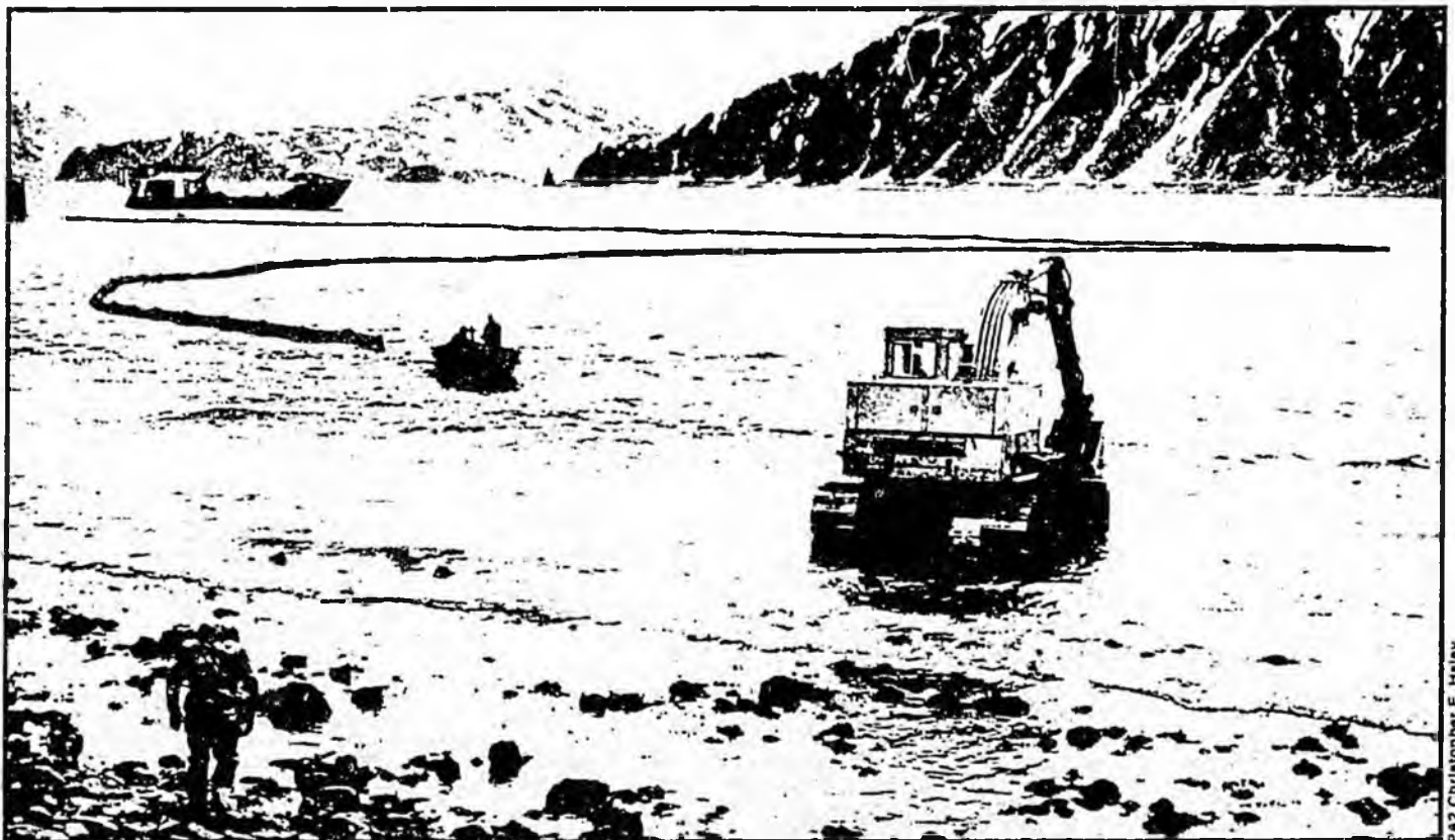
Twelve Hundred feet of containment boom is deployed by Pacific Area Strike Team members and the landing craft Krystal Sea with help from a back hoe.
