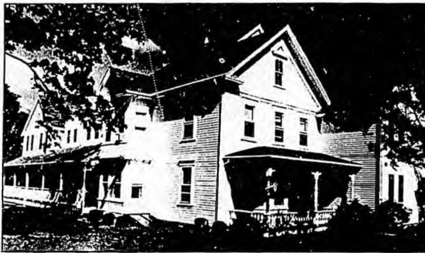
Eldridge House in Hyannis, Mass. (Photo by Mark Cote)
