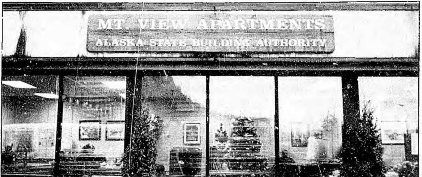
Mountain View Center, Juneau.
