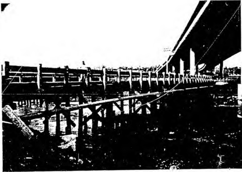
OVERALL VIEW OF BRIDGE LOOKING NORTHWEST.
