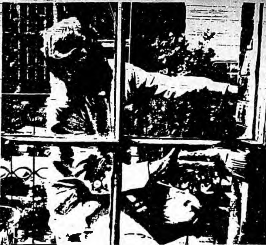
Brush painting is the least hazardous method of application, and because it is the slowest, it is usually reserved for small, inaccessible surfaces.
