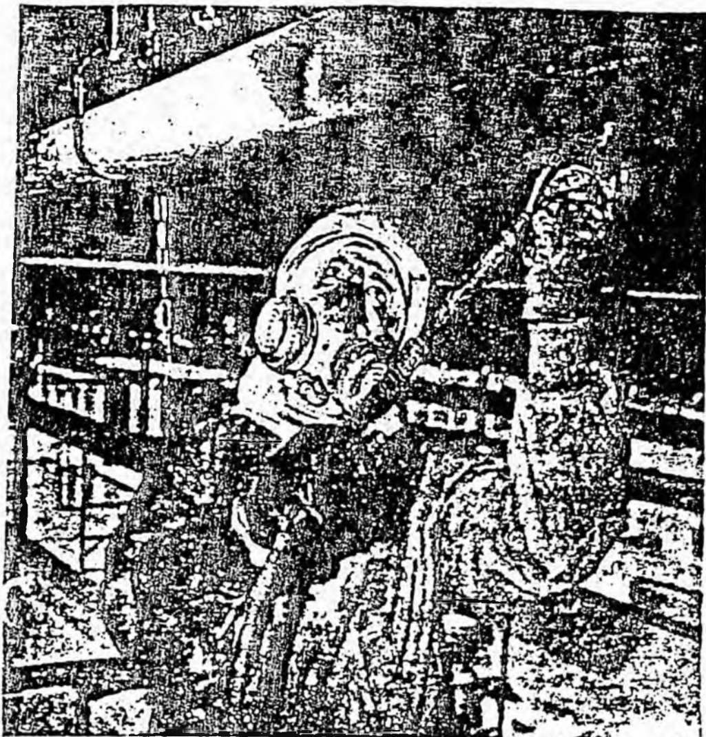
A painter wearing a protective air mask spraying overhead pipes at a construction site on Long Island
