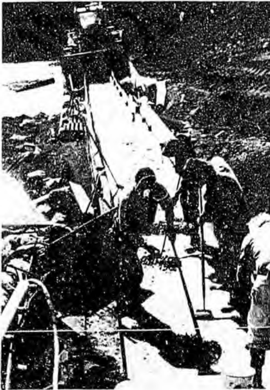
Cleaning sluice box. (PHOTO BY C.B. GREEN)
