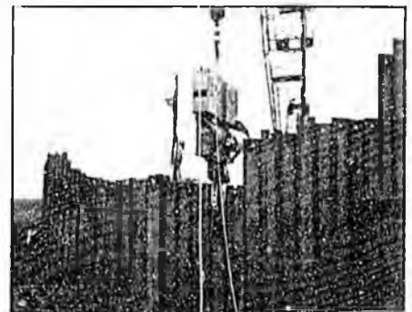
Up to 44,000 sq. ft. of sheet pile will be driven to form open-ended cells and flank walls at the abutments of four bridges. The design provides high load-bearing qualities while preventing fill encroachment into streams. PN&D photo.
