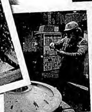
Chris Brooks, a machinist in the Anchorage wheel shop, uses a calliper to measure the axle bore of a wheel.
