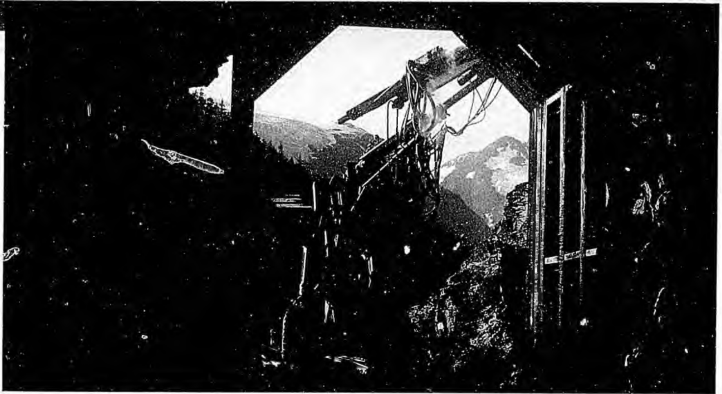
Rehabilitation of five tunnels between Seward and Portage was the single largest track maintenance expenditure in 1985. The $4 million, two-year project will be completed in 1986.
