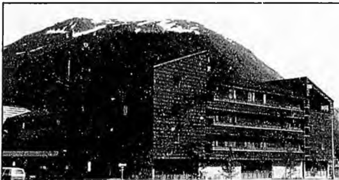
This new addition to the Mountain View project in Juneau added 20 units of senior housing and ancillary facilities.
