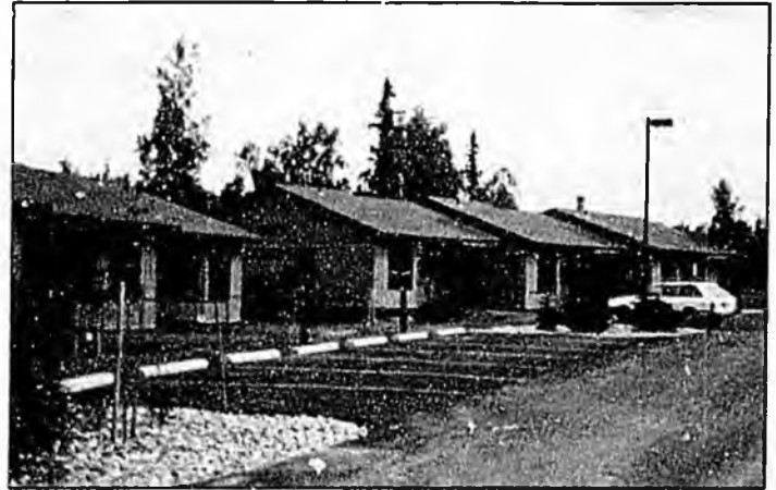
Wasilla senior citizen housing provides 18 units of new senior citizen housing for the Matanuska-Susitna valley.
