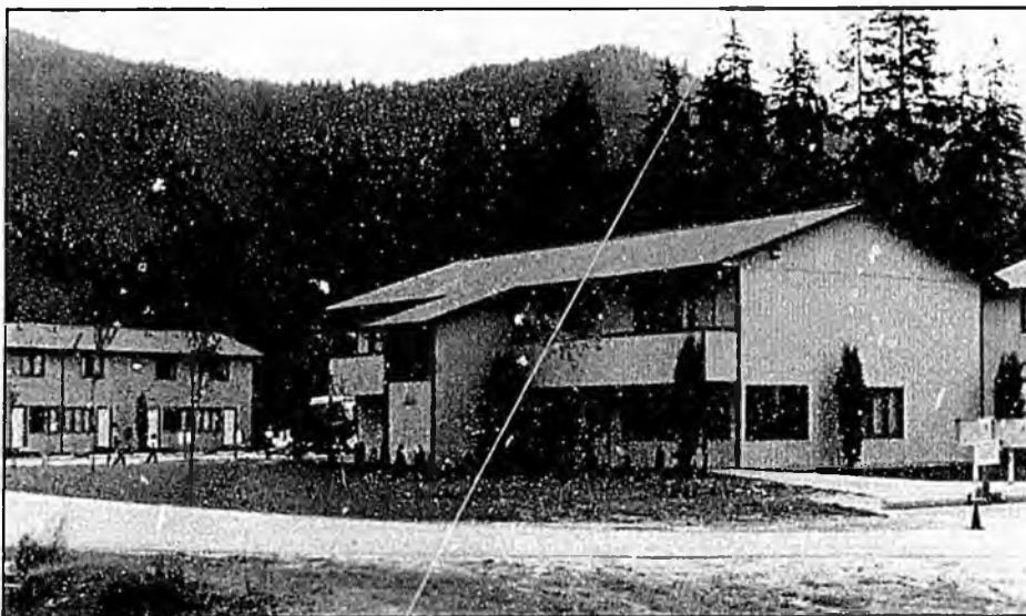
Chinook Apartments 64 one and two-bedroom apartments located in Juneau on a 2.7 acre site.
