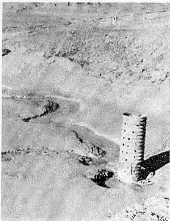
Sediment traps fill rapidly with sediment during periods of construction.
