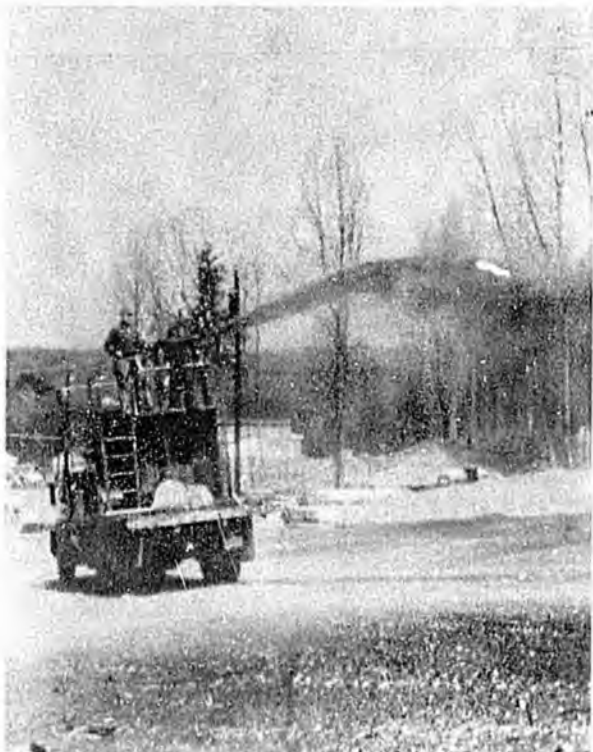
Hydro-mulching prevents erosion of bare soil.
