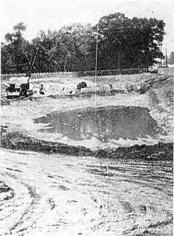
Sediment traps can be used on land undergoing construction to inhibit the movement of sediment to streams.
