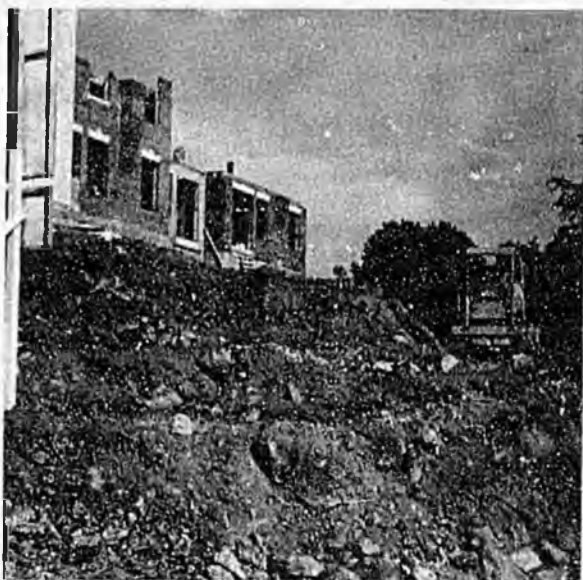
Erosion from bare soil during housing construction is one of the sources of sediment.
