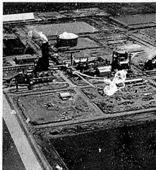
Calgary, Alberta: the Curseland fertilizer \Delta operation is one of Cominco's eight plant food facilities in North America.
