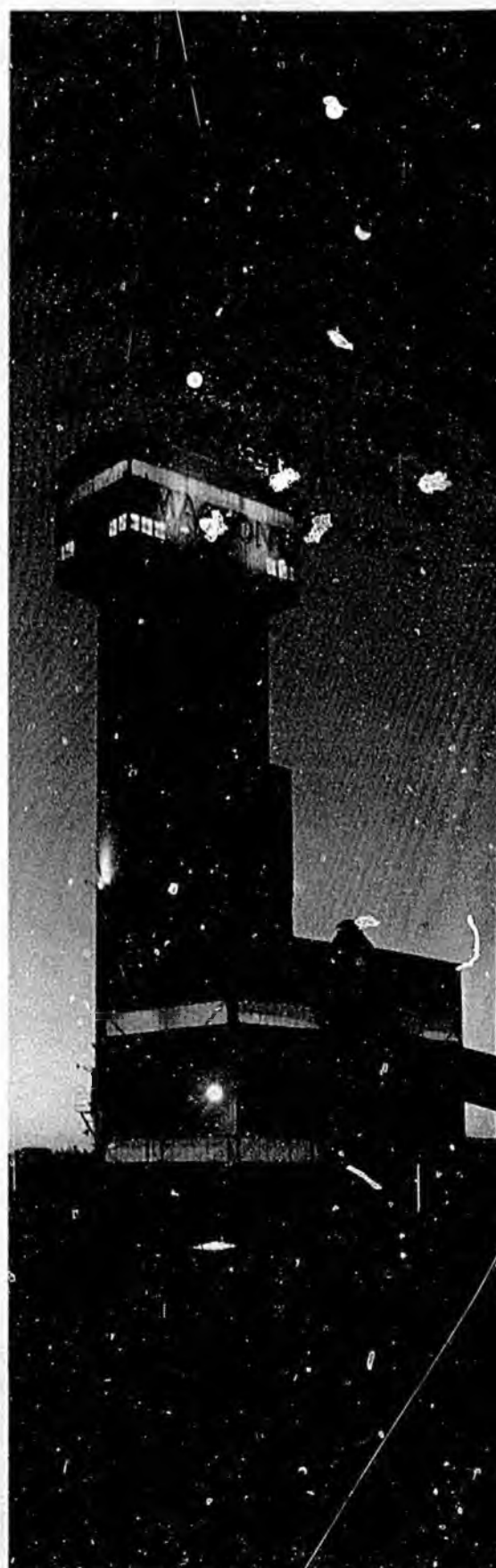
Bixby, Missouri: the headframe of the Magmont Mine.
