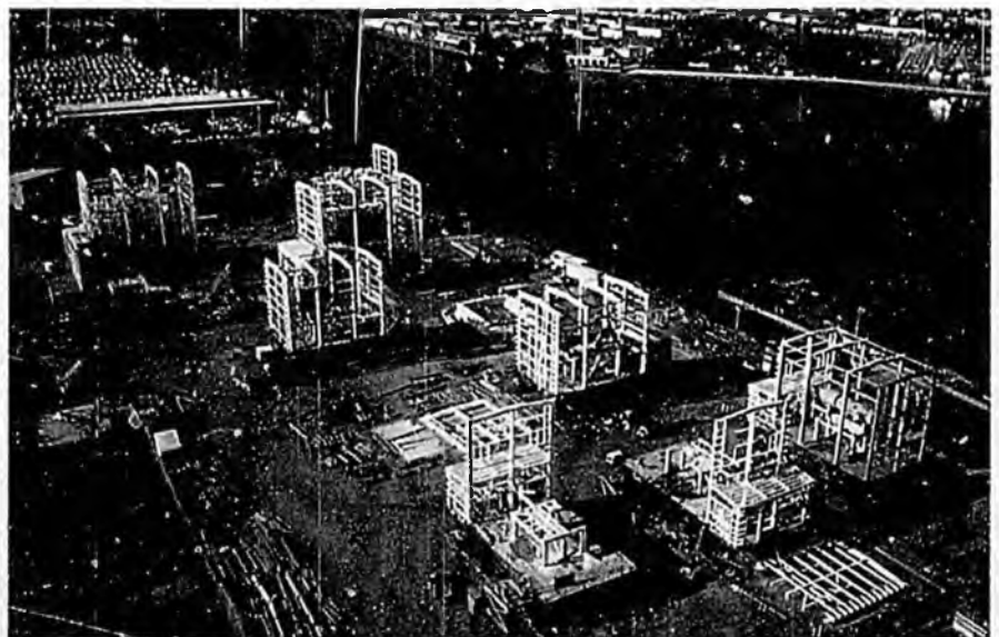
These modules, bound for Alaska, were constructed by National Shipbuilding Company in San Francisco.
