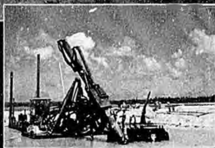
Mataiva: Like the spokes of a wheel, dykes radiate out in this lagoon in French Polynesia, South Pacific. Papeete is the closest town to this joint-venture project, still in the feasibility-study stage. The dredge, left, pumps phosphate mineral samples into the basins formed by the dykes, part of stringent environmental measures.
