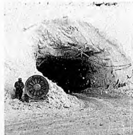
Air conditioning for the Arctic: ventilation fan at the mine entrance.
