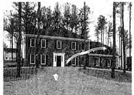
This new Marietta, Ga. home was unoccupied and unheated when temperatures dropped to near 0°F. The plumbing system froze but when the thaw came there were no breaks or leaks in the polybutylene pipe.
