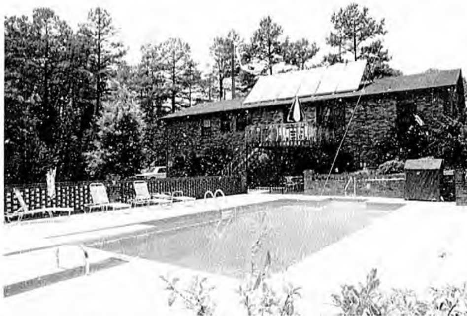
Six south-facing, medium-temperature collectors provide as much as a quarter of a million BTUs a day for domestic hot water, space heating and pool heating.
