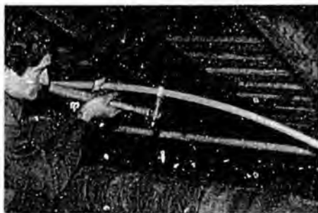
Flexible, lightweight polybutylene pipe helps enable Klein to retrofit an entire plumbing system in half the time required to repair with metal pipe.
