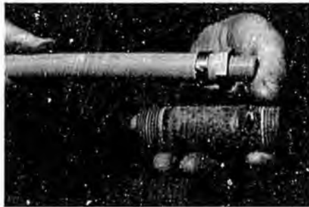
The corroded galvanized pipe (bottom) is typical of the problems Laurence Klein encounters in older water systems in Houston.
