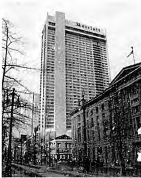
The 42-story Marriott Hotel was the first commercial high rise building in New Orleans to install a fire sprinkler system using polybutylene pipe.
