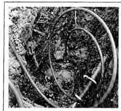
Two lines for separate homes spiral from double strap saddles.
