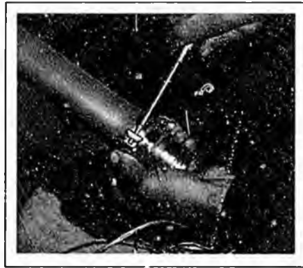
A brass barbed fitting is inserted into the end of a coil of pipe and tightly secured with two stainless steel clamps.
