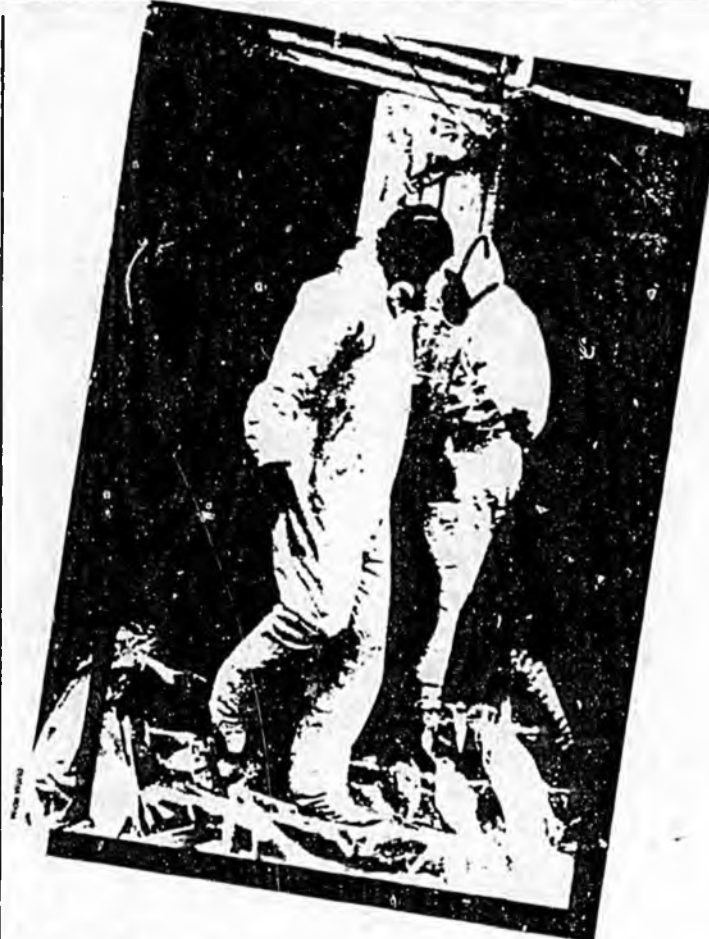
Workers wearing protective clothing and respirators carry bags of asbestos-contaminated materials from a school in New Jersey. Asbestos is just one of the toxic hazards in America's schools.
