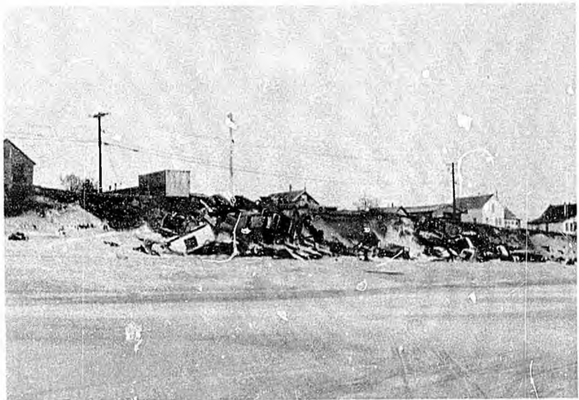
Mission Road area, looking upstream.
