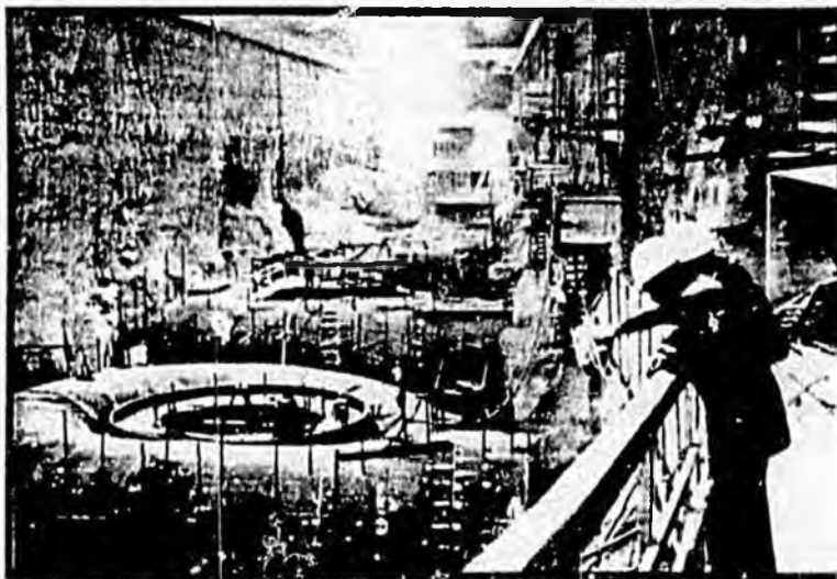
Power from LG 2's 5,328-Mw capacity machine hall was delivered early.
