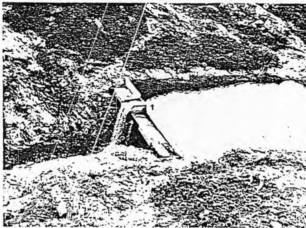
Existing Chester Lake water supply dam. An inspection report favored replacement, and Harza recommended a new concrete arch-gravity dam downstream.
