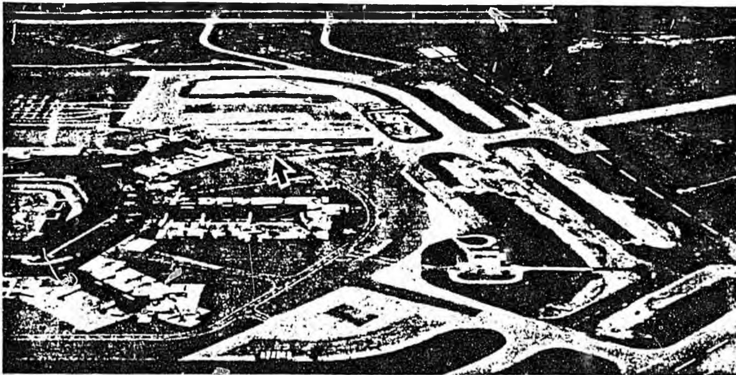
New terminal (arrow), and airfield paving at Baltimore-Washington International are coming in cheap and fast.
