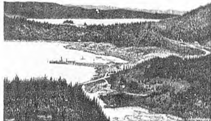
KP 10 Floating construction camp for construction workers at Ward Cove - June 30, 1952
