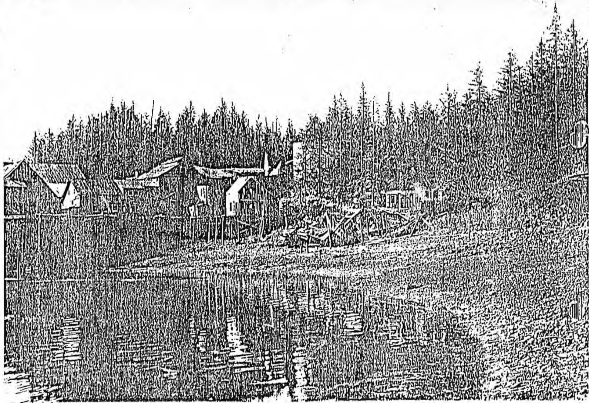
PHOTO #3. Cannery damaged during and abandoned after 1964 earthquake (uplift in area 8 to 9 feet).
