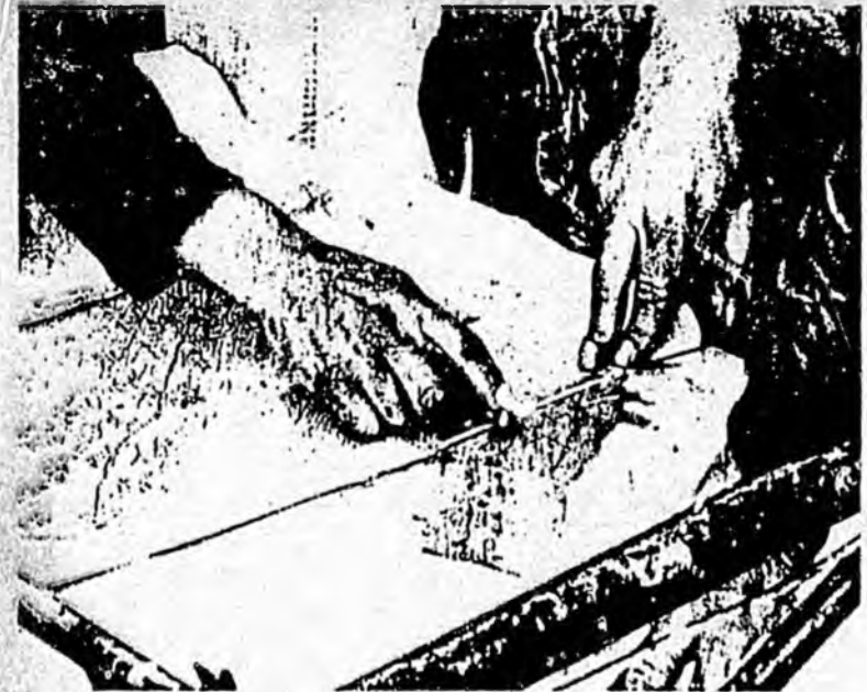
Survey crews locate areas where survey monuments need to be placed so aerial photographs will have ground contact.
